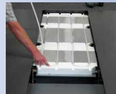
4. Installation of the heating tubes.
