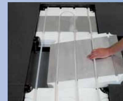
2. Unclip the heating tubes and simply remove insulating thermal unit diagonally upward. Electrical cables are now accessible.
